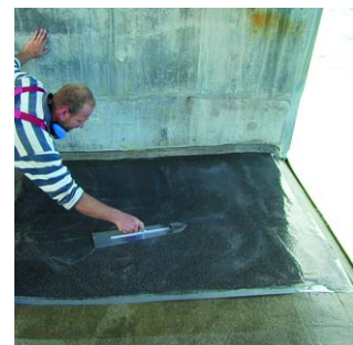
Acrydur® Bridge applied by trowel. It is also possible to install using broadcasting technique.
